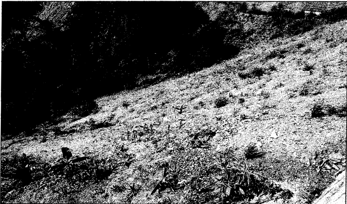
Spoil Bank-10 km 354+450 (Bottom Protection Start Soon)
